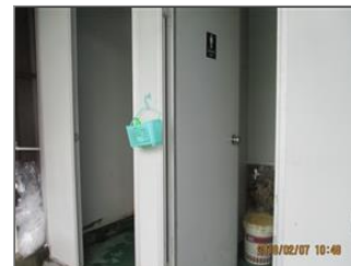
Photo of the sanitary facilities Toilet.JPG
