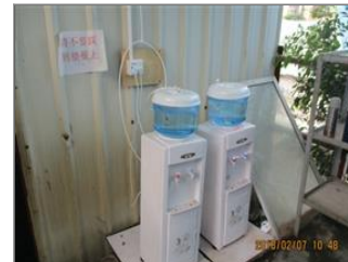
Photo of the sanitary facilities Drinking water.JPG
